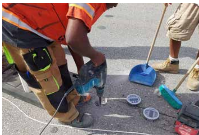
Placing the solar cat's eyes in the Rincon road. Photo OLB
