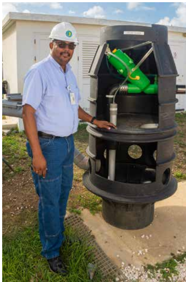
Plant manager Arthur Janga and a life size model of one of the 650 vacuum chambers that move the waste water along the pipeline.
