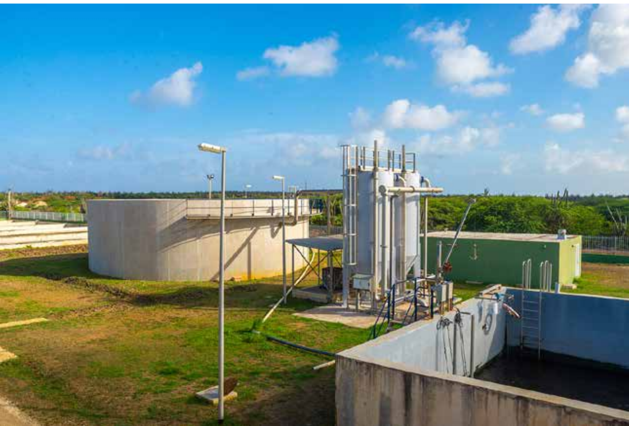
A few of the necessary components needed to turn waste water into irrigation water. L-R: drying pans; storage tank; sand filter silos; UV and irrigation pumping station and storage tank #2.
