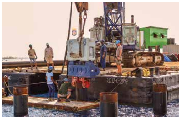
The south pier, previously repaired, is now being extended by 44 meters. The 21 posts that will support the addition have been drilled into the seabed and strengthened with concrete. Early next year, the pre-built parts of the pier will arrive from the Netherlands. With the expansion of the south pier, the center pier will be always available for containers. Both cargo and cruise ships will be able to dock better, as will car boats.
