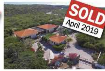
Sabadeco, Crown Shores 59
