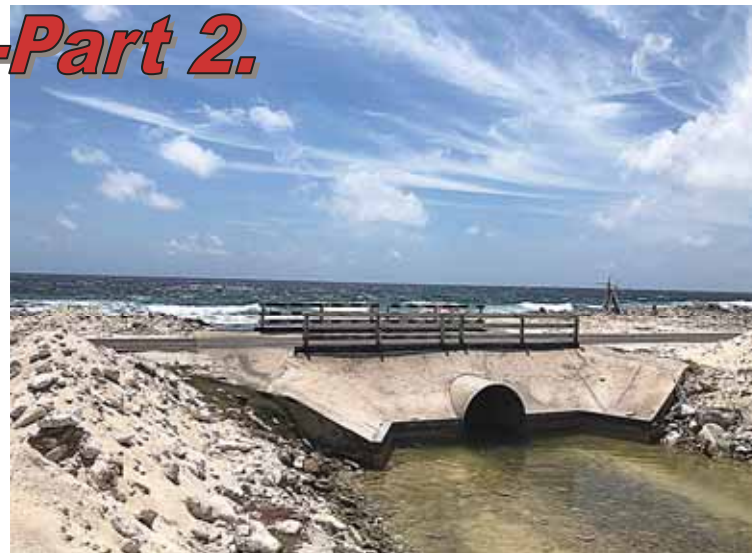
Pipes, as in the south of Bonaire, can open the sea to Gotomeer
