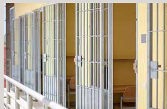
Row of double cell accommodation, air cooled
