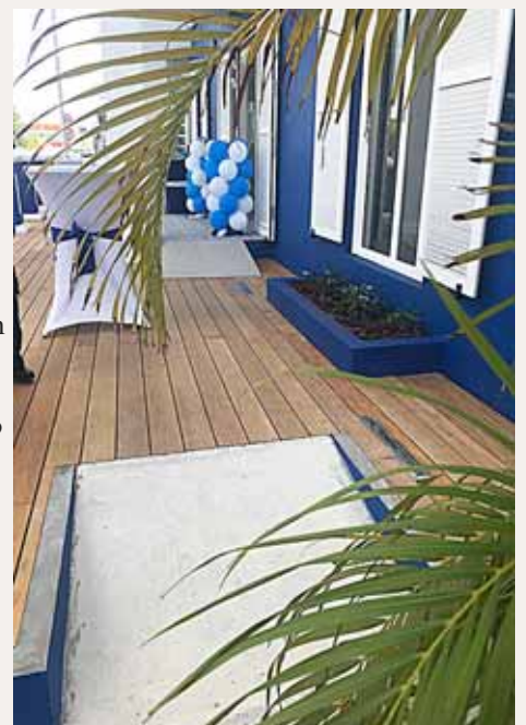
Double ramps at the real estate office make access easier
