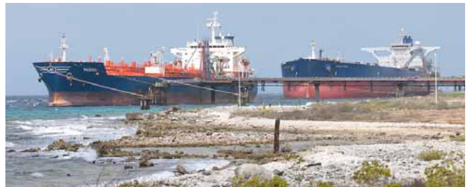
The view of the BOPEC jetties most Bonaireans see. Jetty 1 is one of the largest in the world. It can handle ships up to a Max. DWT of 500,000 tons with a draft of 97' (29.5 m)
