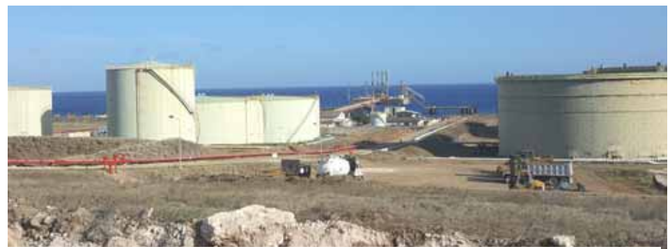
BOPEC tanks are huge. They dwarf the heavy truck at right
