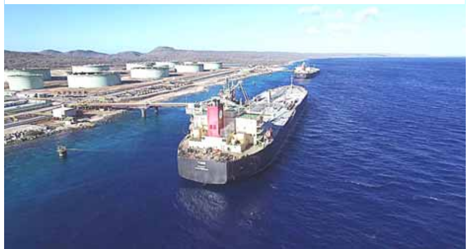
When the BOPEC piers were built they were among the longest in the world
