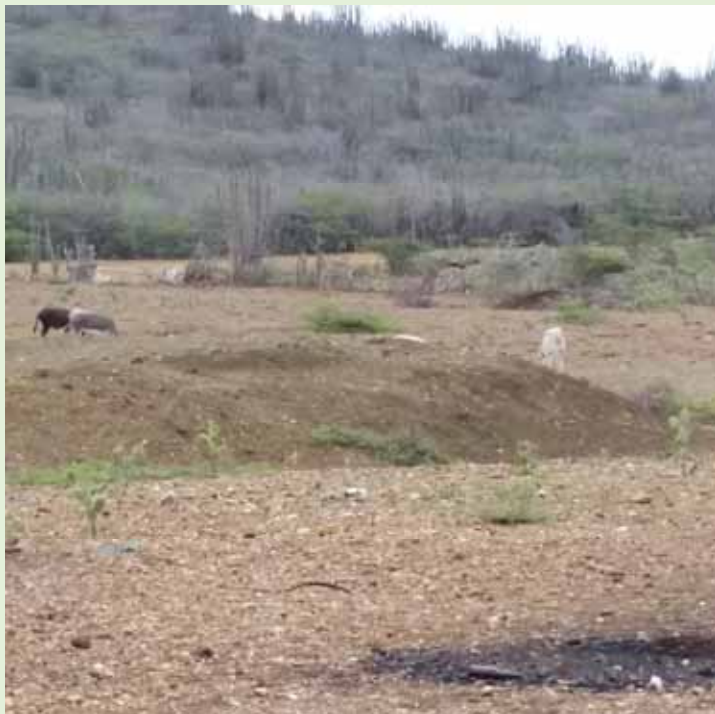
The mound of earth in the foreground, and the depression behind it to hold rainwater is a Bonairean "dam."
