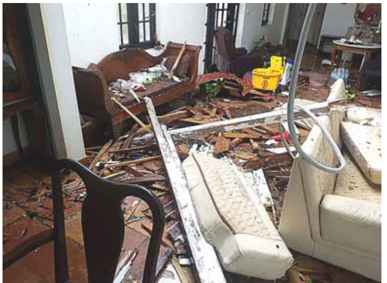
Our roof, our TV, couches, our things—all demolished before the eye passed and it started blowing again
