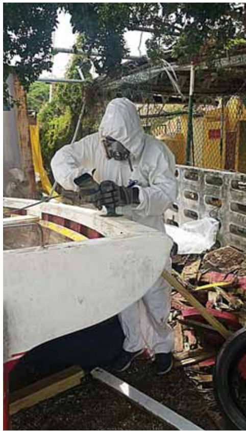
Using modern methods for restoration
