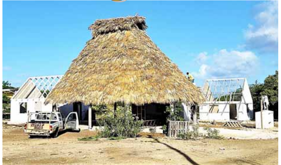
GAZEBO ROOF READY
