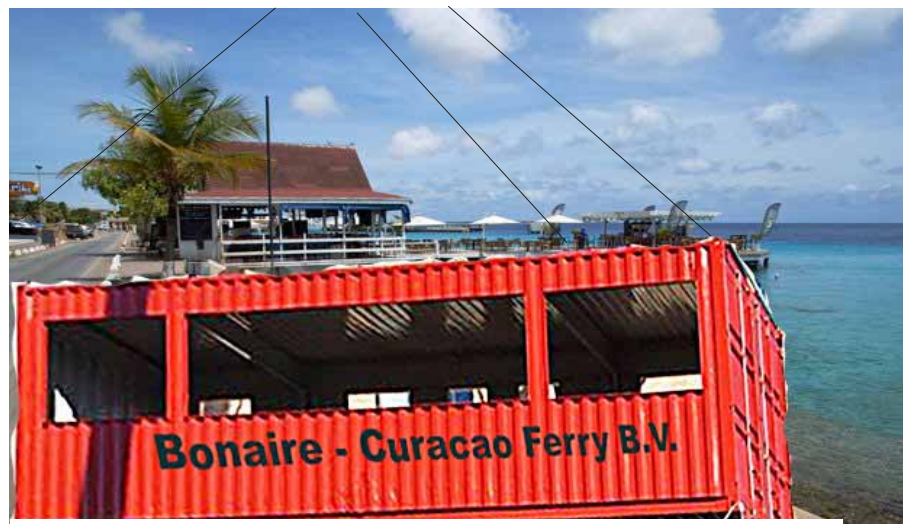
One of the car-carrying containers gets loaded at the waterfront before its windows are installed
