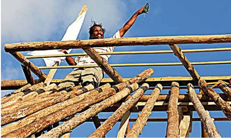
Gibi baptizing the highest point of the structure with a beer
