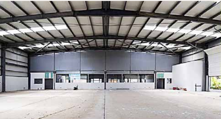
Progress in the construction of the new Bondigro building on Kaya Industria
