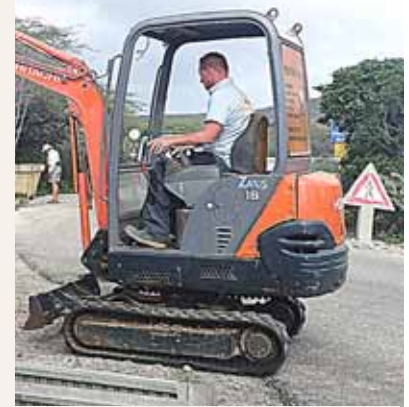
Heavy equipment helped
