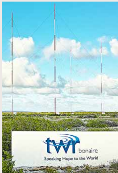
TWR Transmitting Towers
