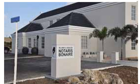
The very attractive office is the new white building is at Kaya Gresia 13, across the street from the RCN.
