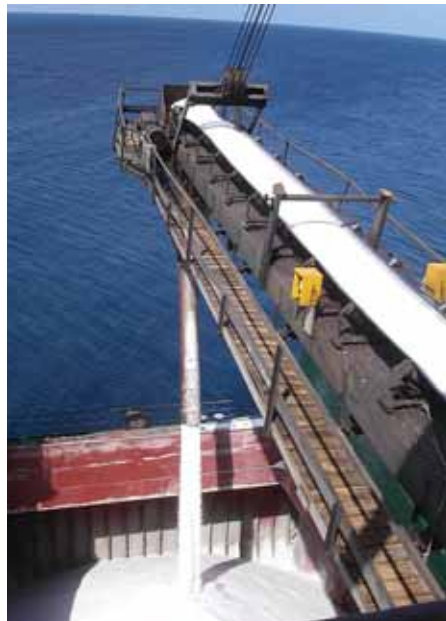
Filling the cargo hold
