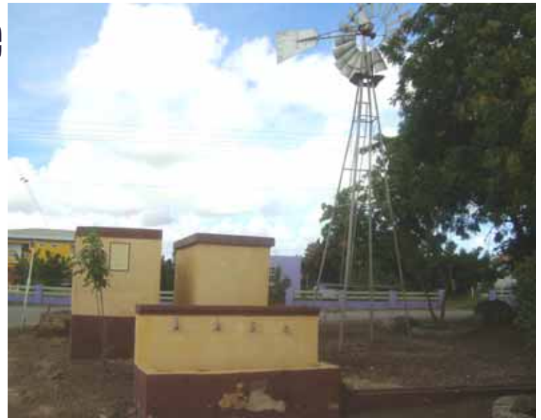
Before the final fix-up, but after clearing the weeds and brush
