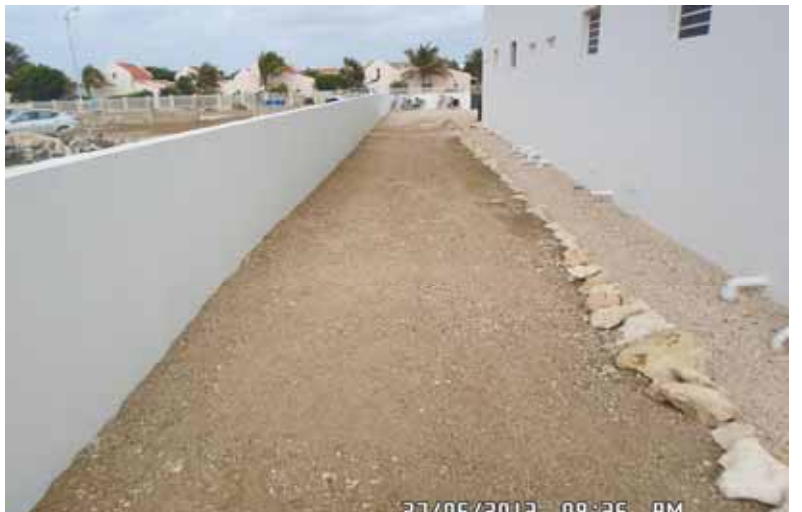
Following the connection, the soil is replace and smoothed
