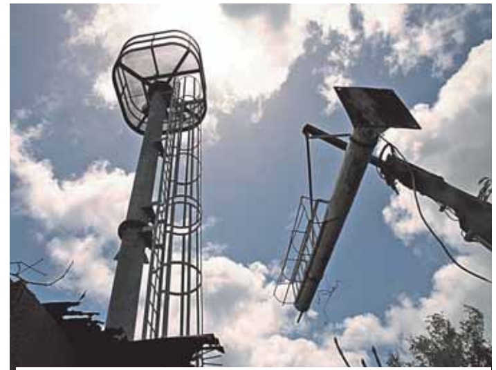
The Wecua Light gets replaced
