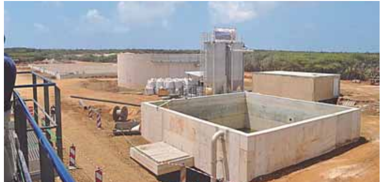
Some of the completed infrastructure
