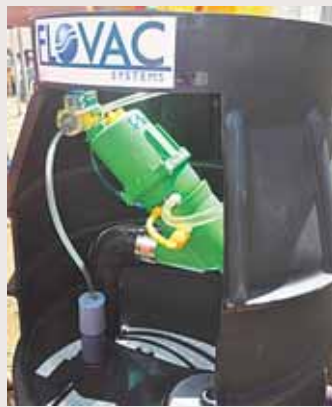
Mechanical vacuum valve
