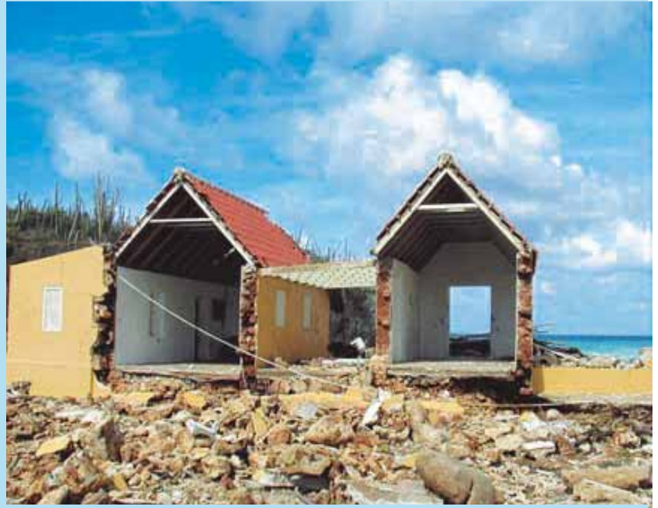
Beach erosion due to loss of shallow reefs leaves historic plantation buildings like those of Washington Slagbaai Park vulnerable. In 1999 waves from distant hurricane Lenny devastated the plantation complex and it had to be rebuilt.
