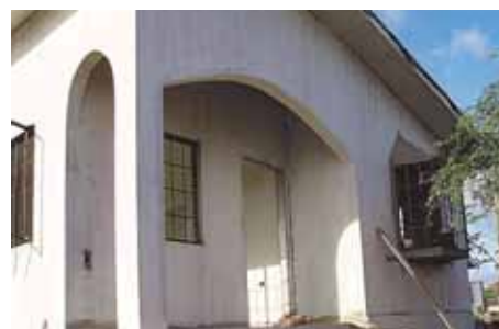
Affordable home under construction
