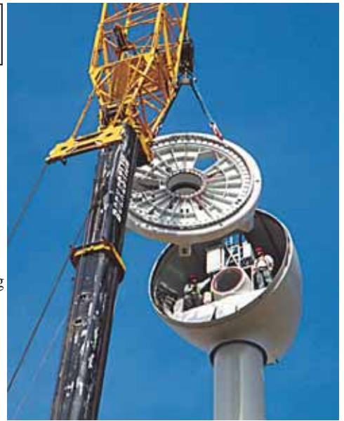
The size of wind turbines dwarf the men installing the equipment.
