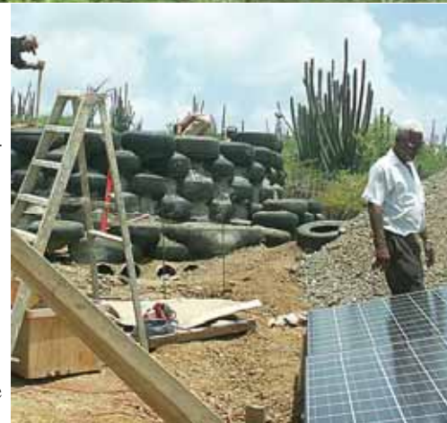
Bonaire builder Sidney Manuel checks out the solar panels
