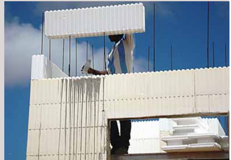
Concrete filled foam blocks make the walls
