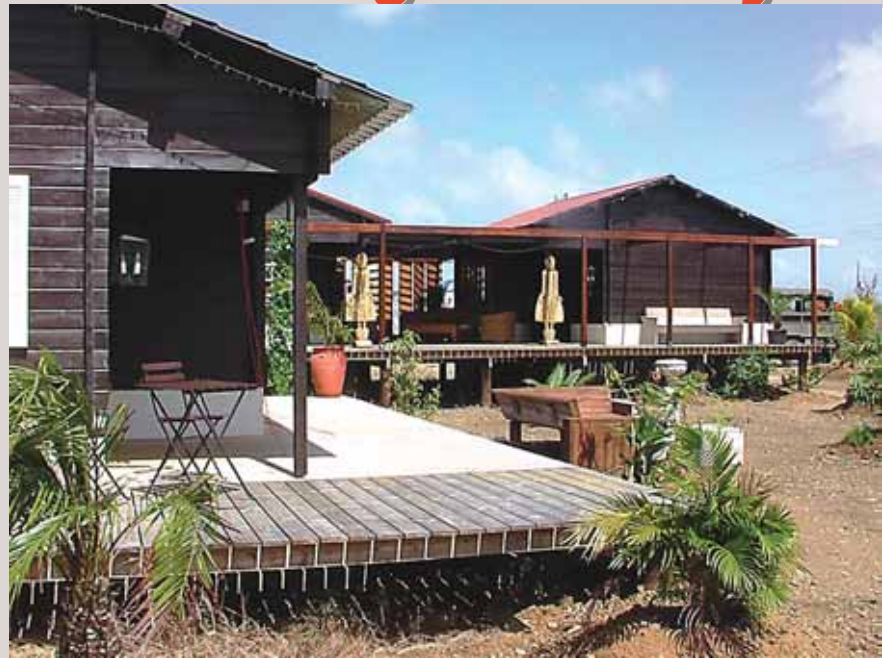
The wooden cottages at Bamboo Bali
