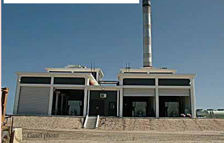
Present WEB Power Plant in Belnem
