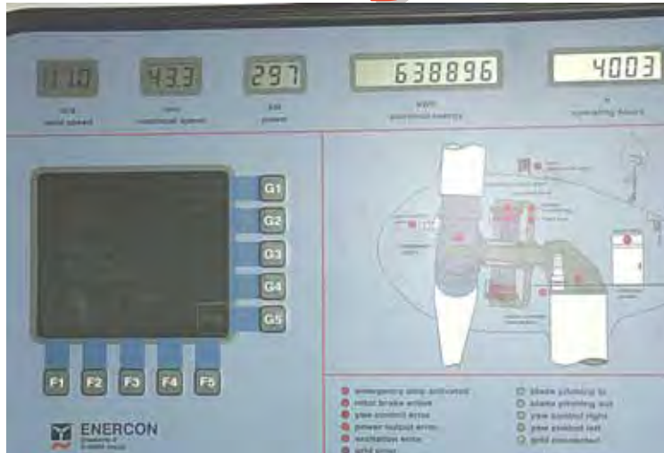
The power panel of the Sorobon wind turbine shows it's producing 297 kW of electricity (enough for about 100 homes) in 20 knot winds. The Morotin turbines are three times more powerful. It has run more than 4000 hours with better than 90% availability.
