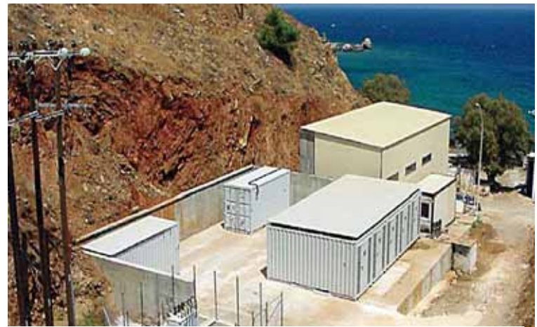
A packaged desalination plant, similar to this, may be installed at the current WEB power plant site after the new facility is operating near BOPEC.
