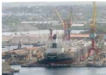
CDM Dry dock
