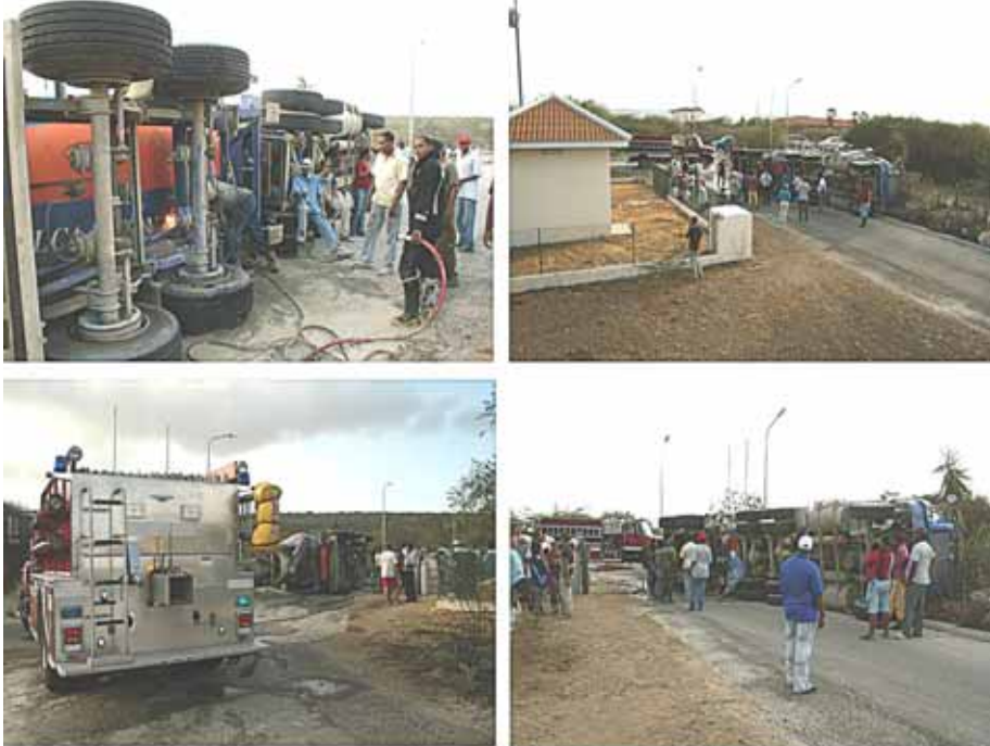
Concrete Spill at SABEDECO photo montage by Sam Williams
