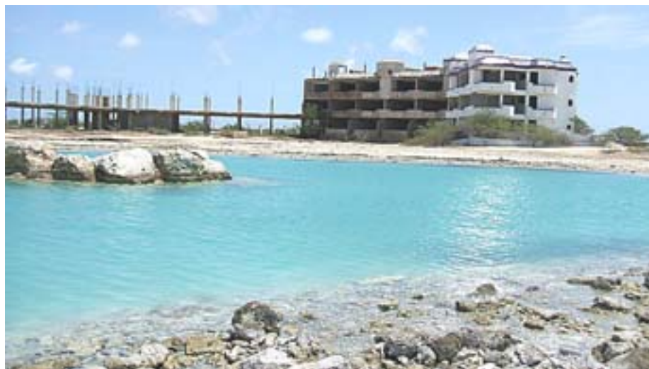
The unfinished Esmeralda Hotel on Bonaire’s southeast coast photo by Jiri Lausman
