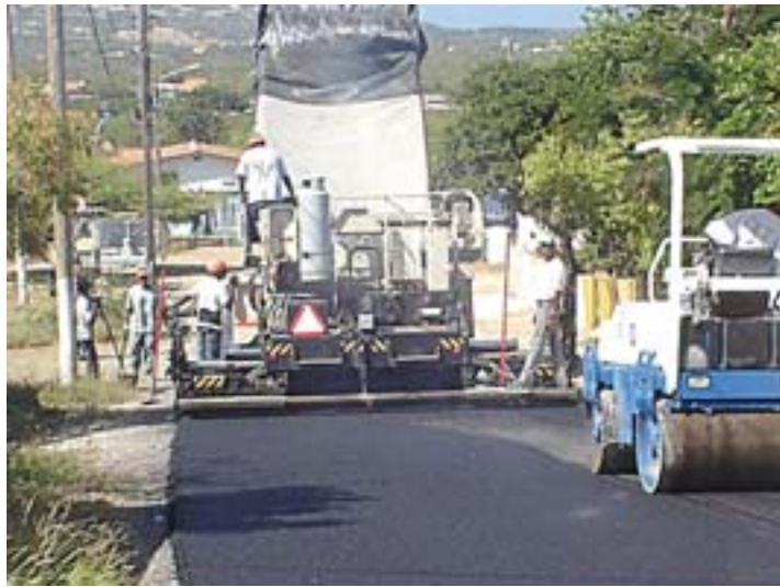
The paving machine in action
