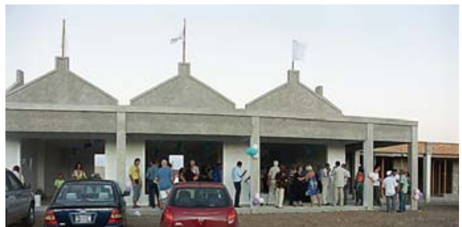
The first buildings are nearing completion. Opening is planned for July 2007
