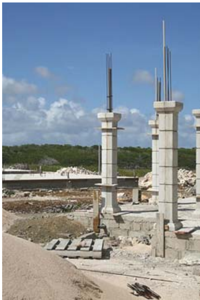
These Mangrove Village columns to be demolished
