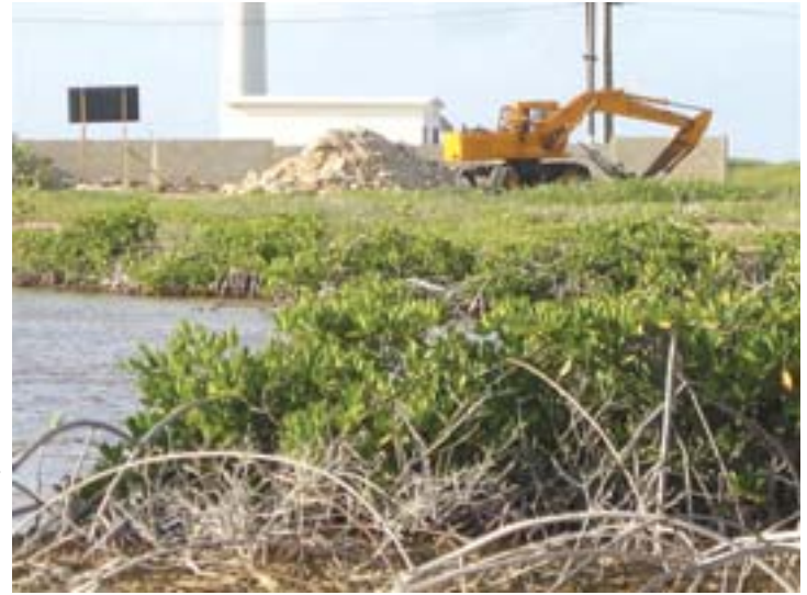
Mangrove Village construction STINAPA Photo
