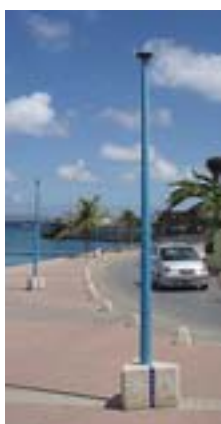
A string of non-working street lights
