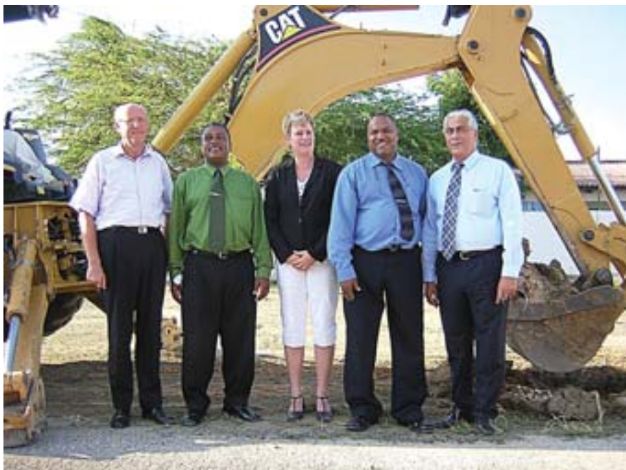
On hand for the ground-breaking were Onno Koerten, Dutch representative to the Netherlands Antilles; James Kroon, Bonaire Commissioner of Sports; C. Ross-van Dorp, Dutch Minister of Sports; Onni Emerenciana, Bonaire Commissioner of Economic Affairs; and Governor Herbert Domacassé
