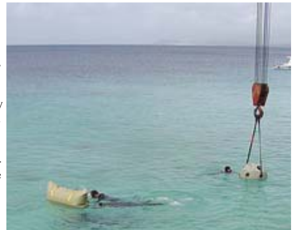
The lift bag transported the balls from the crane
