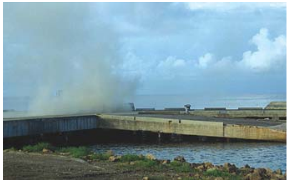
Clouds of cement dust raised during the cleanup
