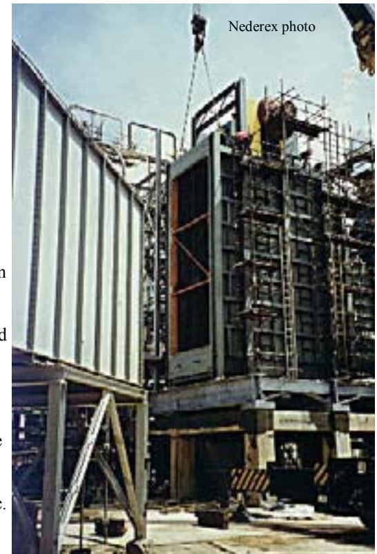
Replacing the troublesome Cat Cracker at PDVSA’s Curaçao island refinery
