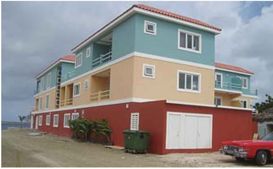
The apartment accommodations built on the site of the Den Laman Restaurant is about to have a Grand Opening. It was built by local companies and labor.
