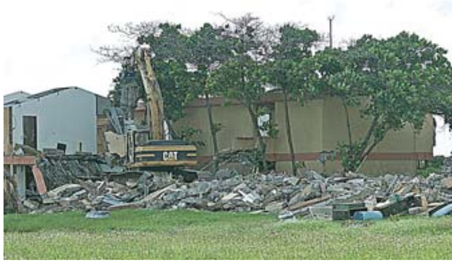
The demolition of Sunset Beach — to be replaced with what?
