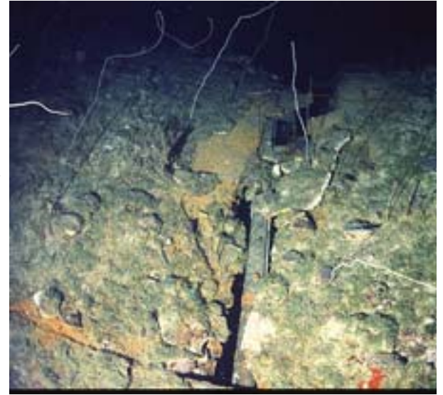
This photo taken from outside the hull shows the expanded crack. Note the rivets popped from the thick hull plates and the bare metal exposed where the coral sheet slipped off.
