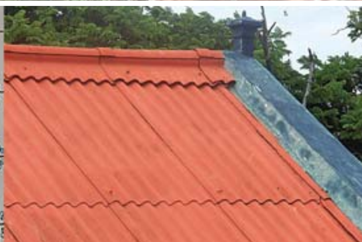
"Builder signed" roof design
