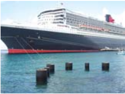
Five of the "dolphins" that were installed at great expense to secure the QM2.
