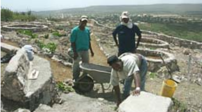
Ruthsel, Jopi and Tico at work on Alta Mira construction
